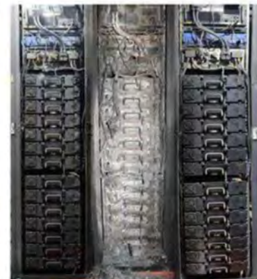
Rack 17 Rack 15 Rack 13
